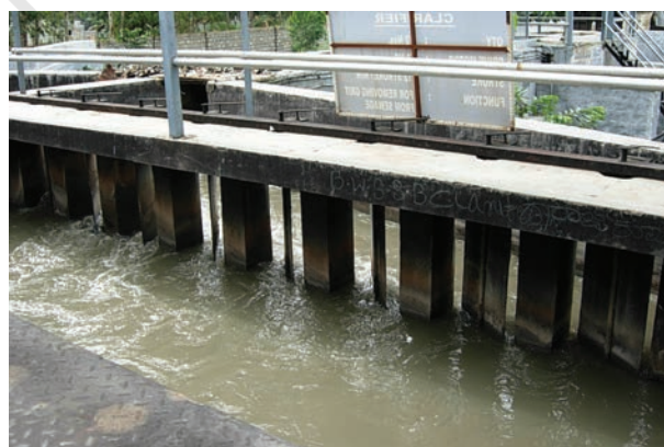
Fig. 18.4 Grit and sand removal tank
